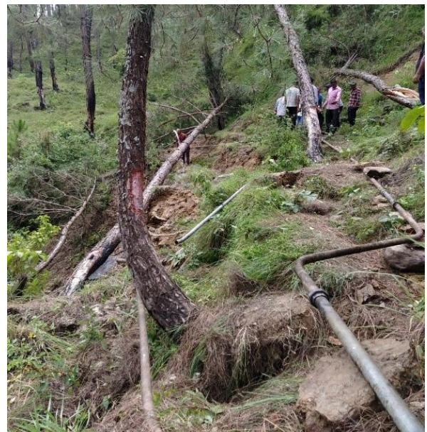
(Damaged pipeline due to landslide in Uttarakhand; Photo: HNBSU)
