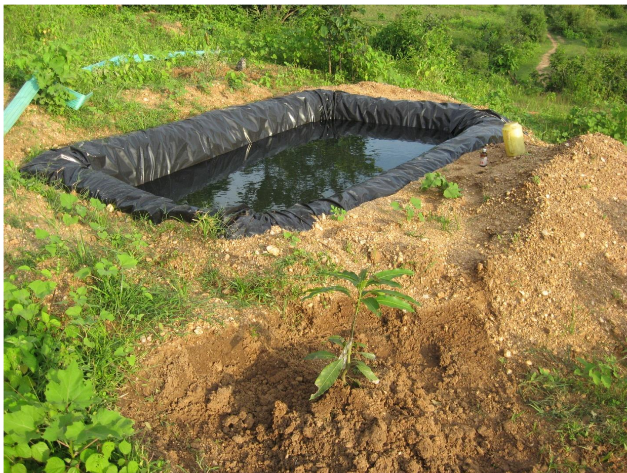
(Poly tank are the low-cost and easy to construct water harvesting structures-. Photo courtesy: Dr. B.P Bhatt )
