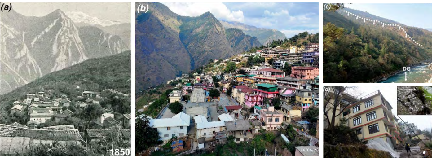
Fig. 5.1: Photos of the Jashimath town (a) in 1850 A.D. and (b) at present. (c) Zone of road subsidence marked in August 2022 and (d) cracks in buildings and roads developed due to subsidence January 2023.
